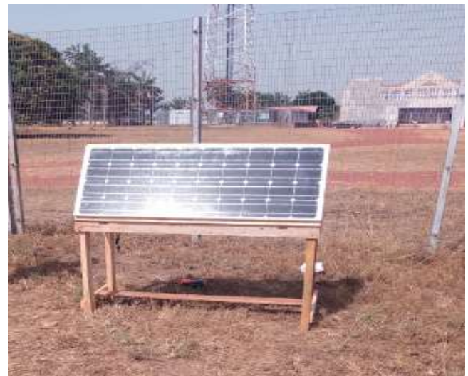
Figure 1: Solar panel on an erected wooden rack.
