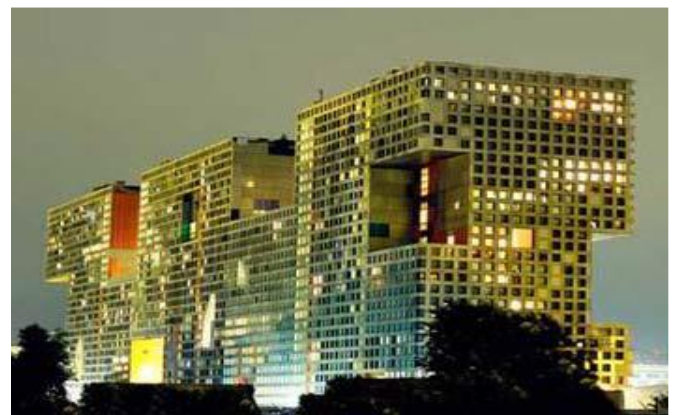
Plate 1: Simmons Hall student residence at MIT showing pores on its facades
